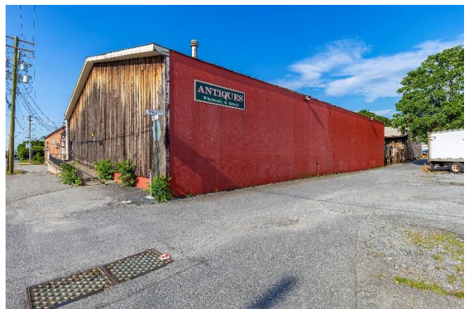
Side View of Warehouse
