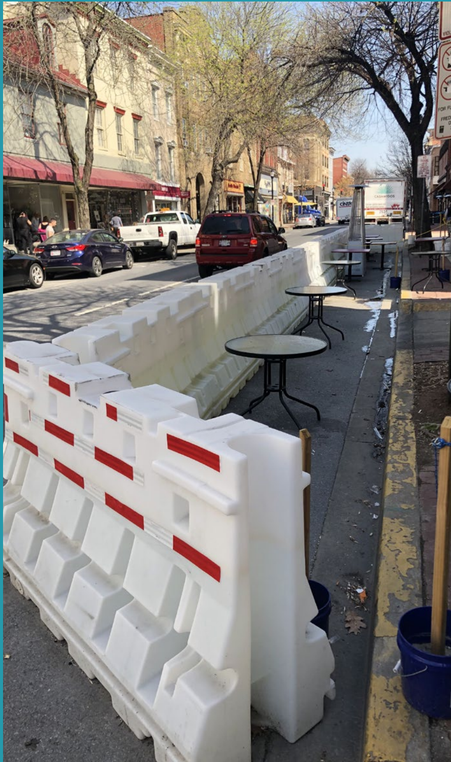
Downtown Frederick - Temporary Water Filled Barriers Source: Design Collective
